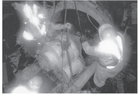
写真-21 ギヤボックス立坑へ
